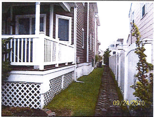
Right Side View – Date of Photograph: (See Photo Stamp)
